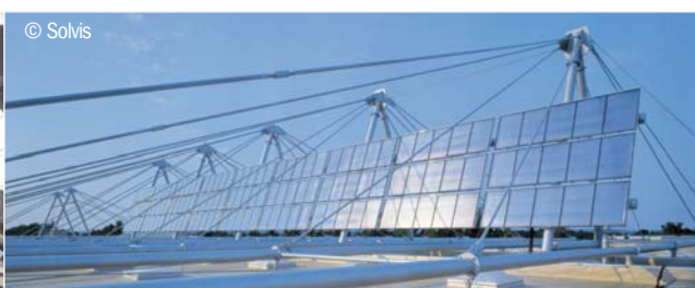
Zero-emissions factory with 200 m 2 roof solar collectors
