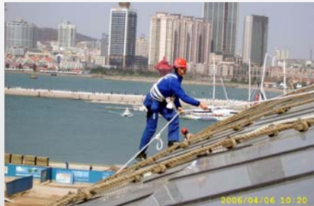
Collector mounting for a Solar Cooling Plant in Qingdao, China, 2006
